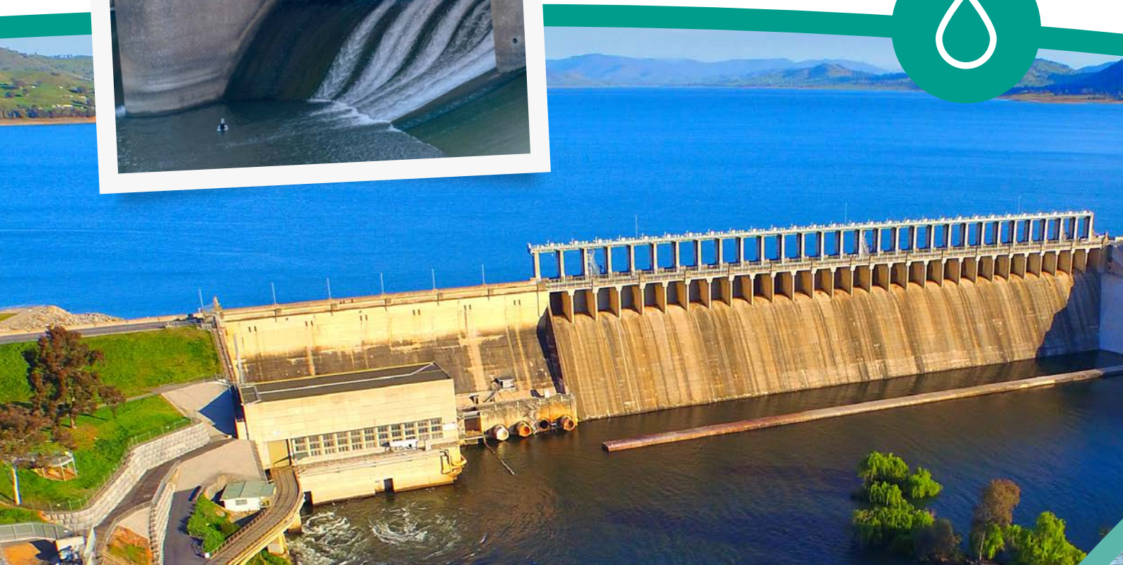
▼ Lake Hume, hydroelectric generator on left of the weir.
